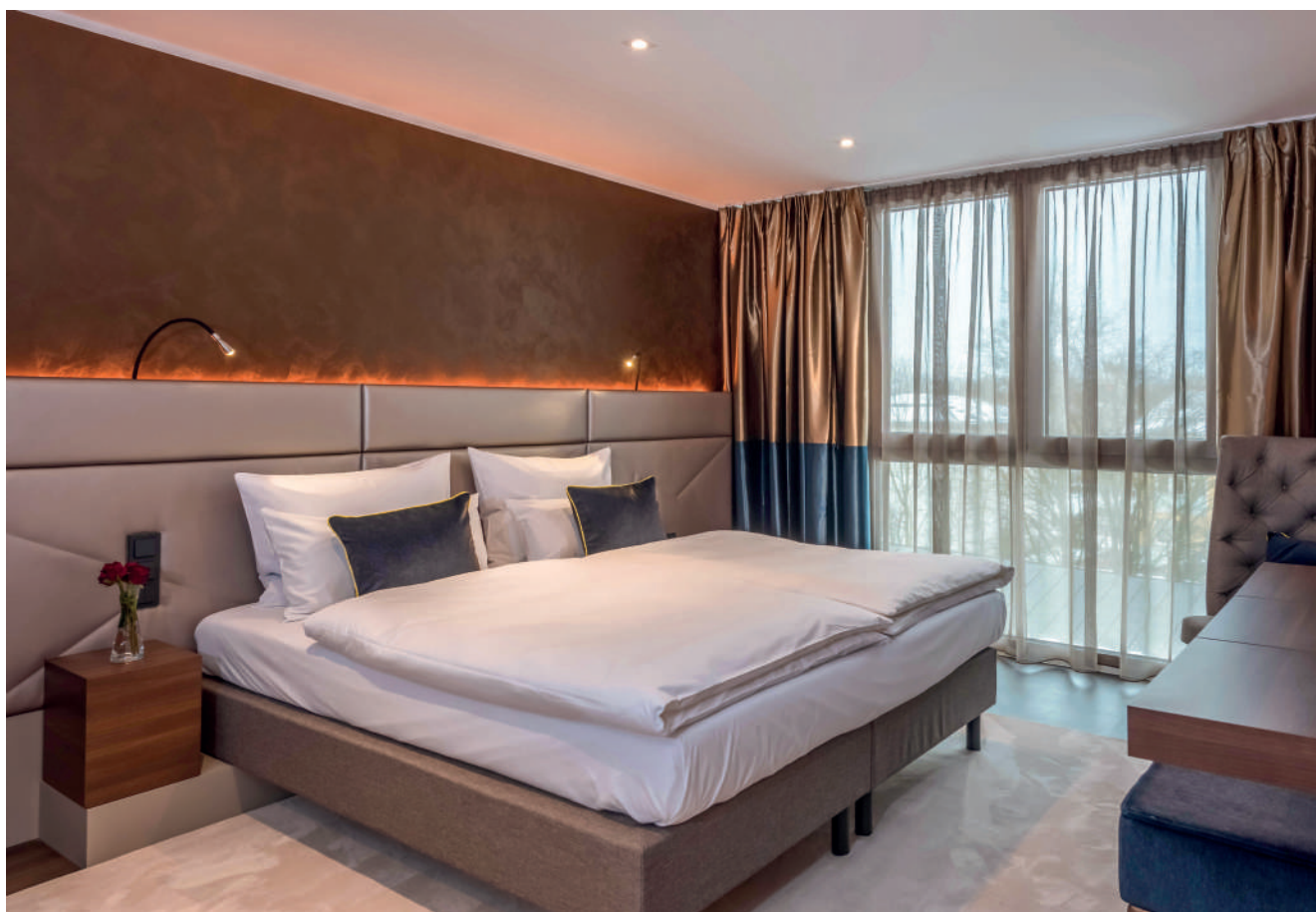
LED downlights provide the basic lighting, the backlighting of bed and television with QualityFlex® ensures a pleasant atmosphere.
